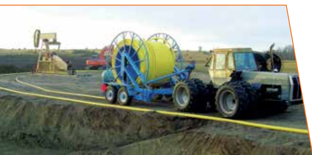
example of application: glassfiber reinforced PE coil tubing
